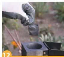
12 Discharge the igniter powder on the thermoweld powder.
