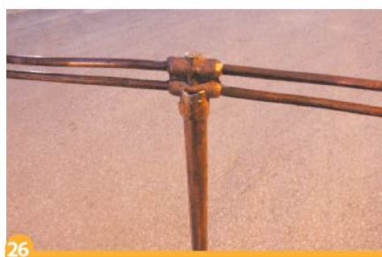
Welded earthing conductors and earthing electro.
