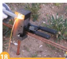
18 It has passed to reaction with high temperature.
