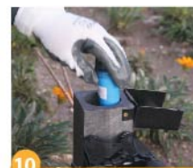
10 Discharge the thermoweld powder into the mould.
