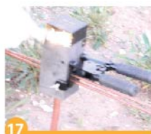
17 Thermoweld powder fired.
