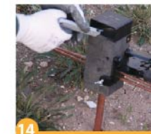
14 Fire the thermoweld igniter by the ingiter gun.
