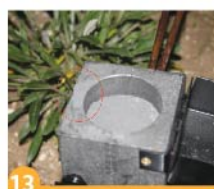
13 Thermoweld system is ready for fire.
