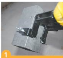
1 Connect the thermoweld mould with thermowelding plier
