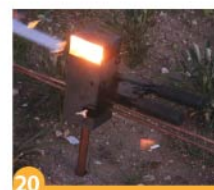
20 Thermowelding has finished
