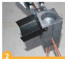
2 Insert the copper wire to inside of the thermowelding mould and put the earthing electro to down side of the mould
